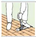
Fit the last row of parquet in its place using the pull iron. The spacers have to be inserted by the wall here also. A 1-2 cm expansion joint also has to be left at thresholds and heating pipes. The installed parquet must not directly touch any wall or other structure of the building.
