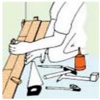
Never rely on the straightness of the wall. Check the straightness of the row using a thin strung thread. Start the second row with the parquet left over at the end of the first one.
